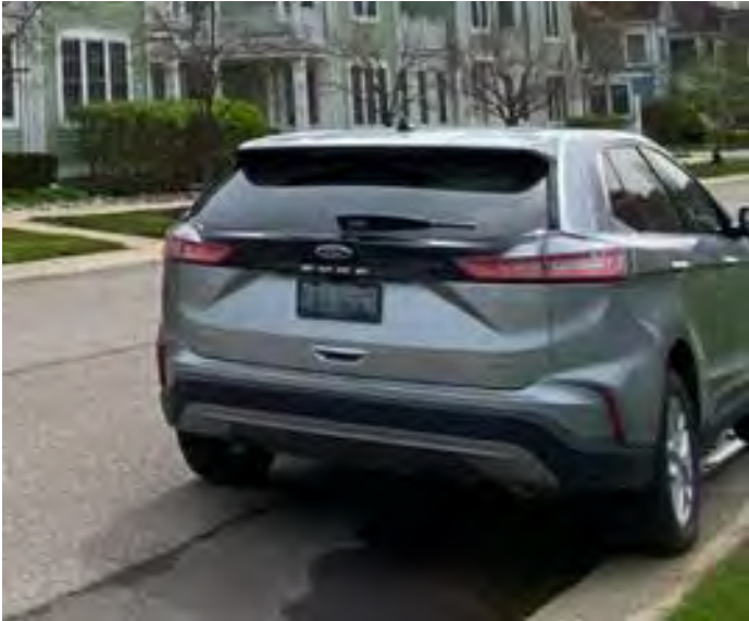
Rolled Curbs allow vehicles to park on curb vs. 6" raised curb
