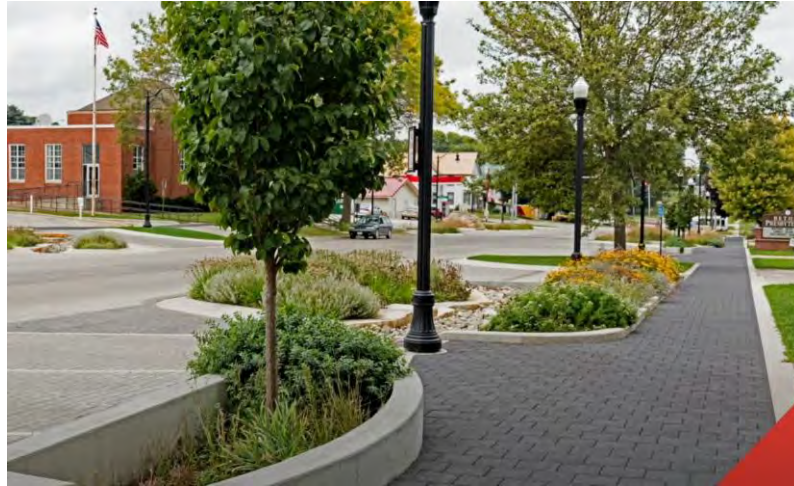
Permeable paver road & pathways
