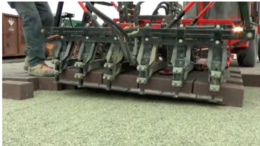
Mechanical rolled and large-scale installation
